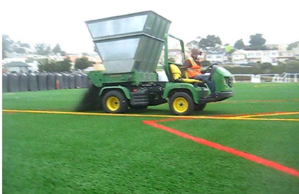
Figure 3: Smaller operations of infilling
