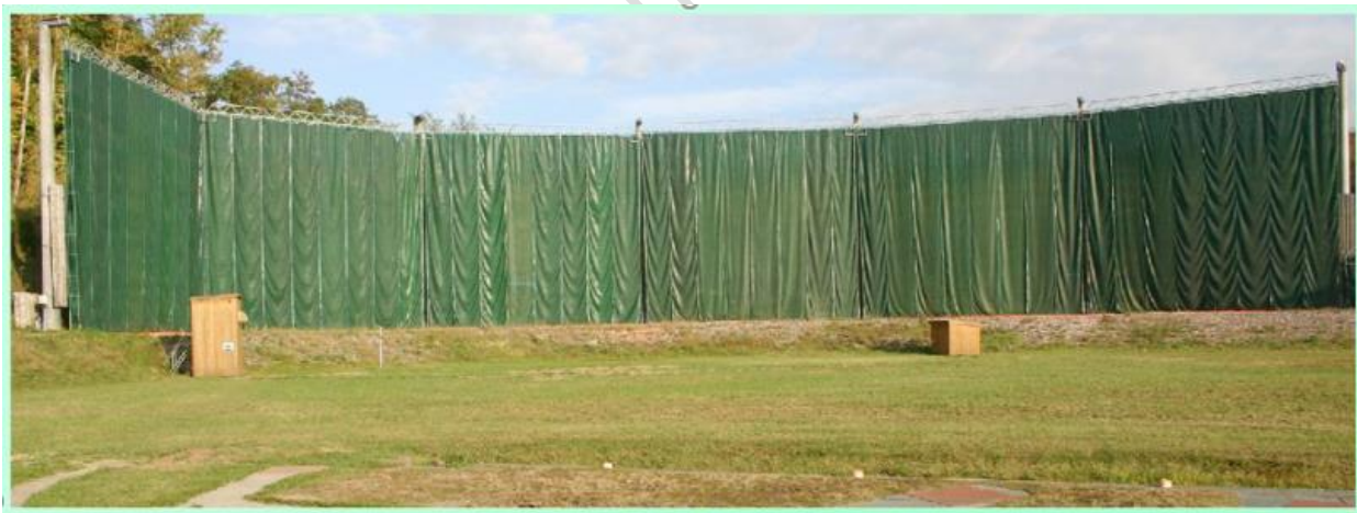
Figure 1-3 Example for a vertical barrier in a clay shooting range (Herrmann, 2013)
