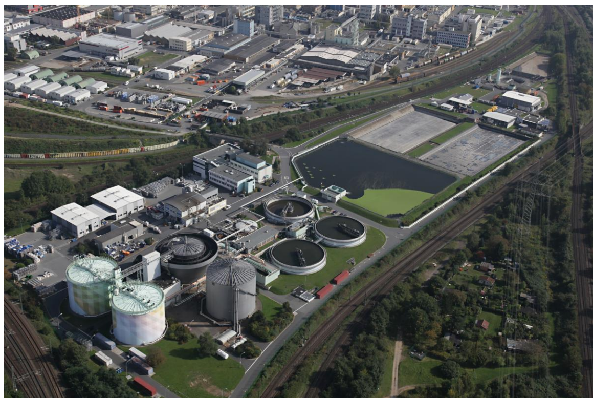
Figure 7: Sewage treatment plant at the Merck production facility in Darmstadt (Germany)
